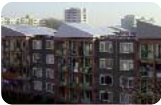
"2 MegaWatt" Project - Netherlands
